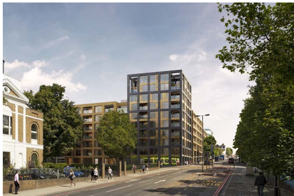
Groverworld & PTE - Pentonville Road, Islington
