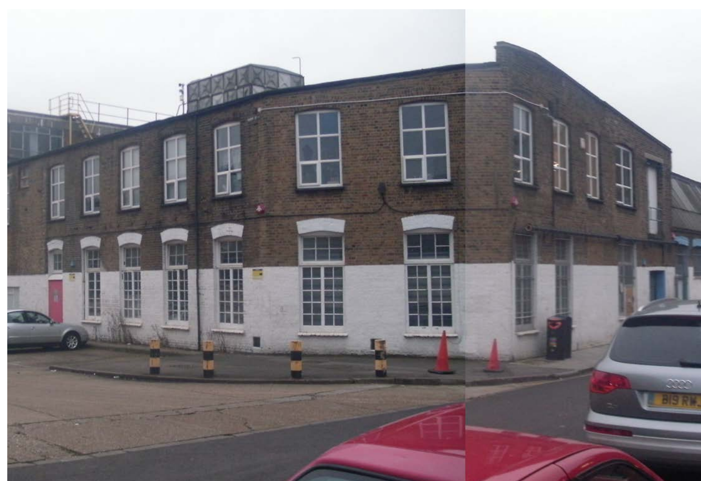
View from Main Yard Wallis Road junction of existing corner building
